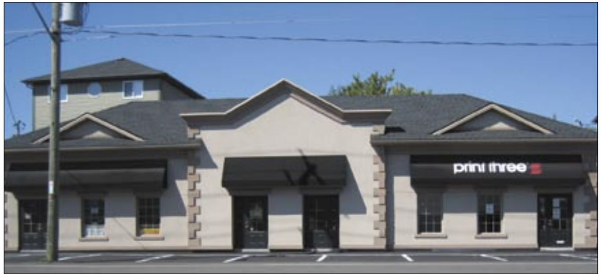
Print Three is a new business owned by franchisee Bill VanderKlippe in Thorold at 15 Towpath Street in a historic building with a new facade. The Towpath Square development by Serge Carpino enhanced the heritage theme in the downtown business community by participating in a facade grant program with the City of Thorold and the Niagara Region.
